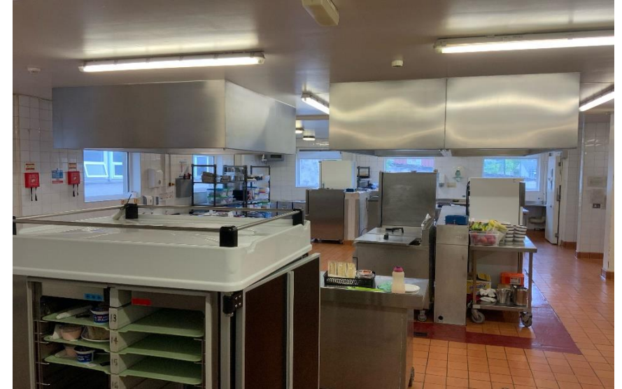
Above: The current kitchen area at Belford Hospital
